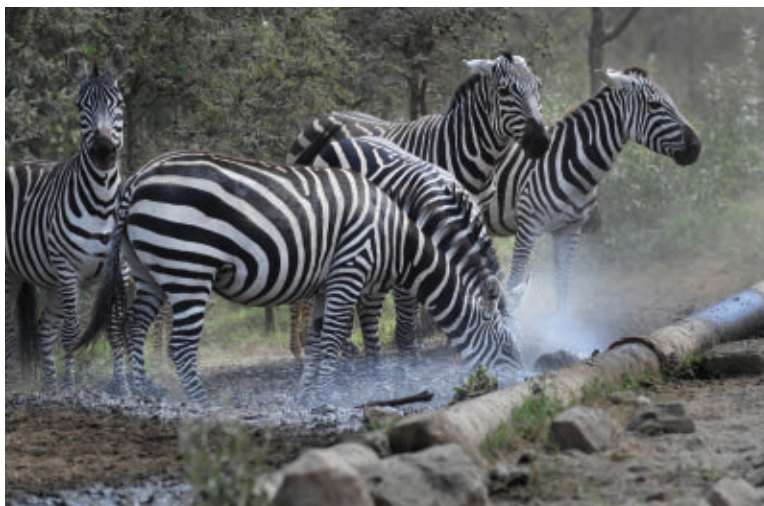
Zebras gather near a tube carrying water that will be injected back into geothermal wells near Olkaria.
