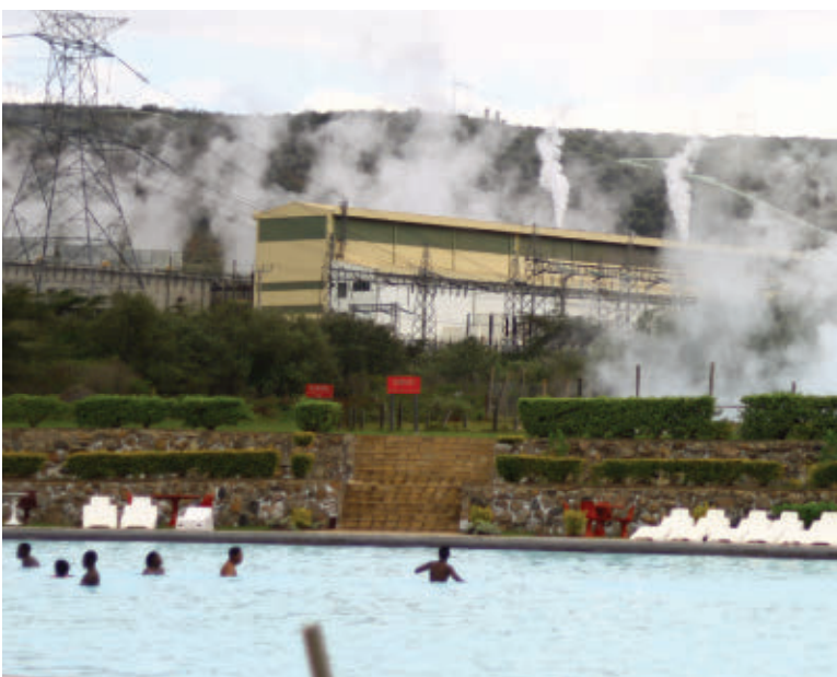
Geothermal energy doesn't just generate electricity. It can also be used as a direct source of heating, like at this spa next to the Olkaria geothermal power project.
